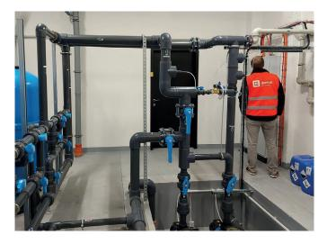
The heat and cold source is a system of heat pumps, supplemented by 300 kW cooling units. Heating and cooling water is accumulated in two tanks of 1500 I and then further distributed to two heating and two cooling circuits. The regulation of individual rooms is represented in the offices of eleven FCU controllers, which control fans and six-way valves for heating and
